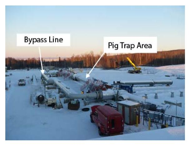
The section of pipe at Pump Station 8 in which the northern PIG was trapped [on the right] and the bypass line (on the left) through which oil is being diverted around it (Photo Date: 1/12/2011).
